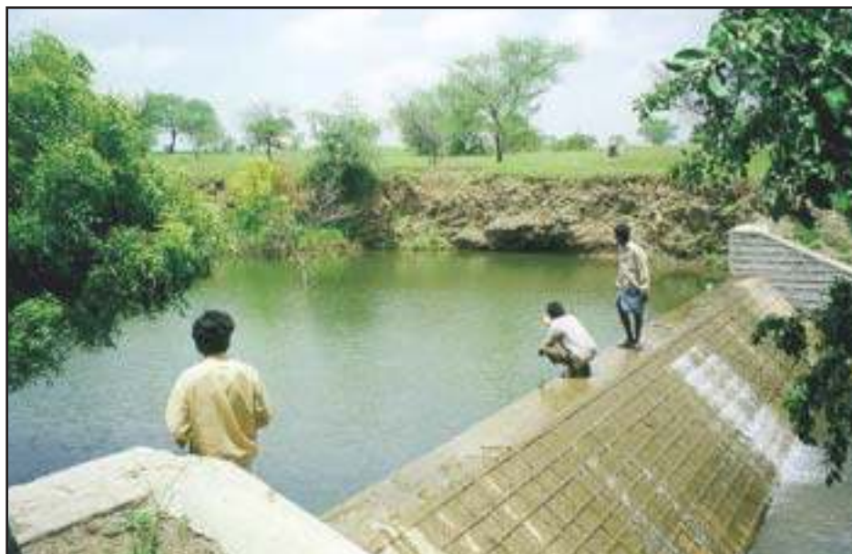
Figure 2. Community-based masonry check-dam.
